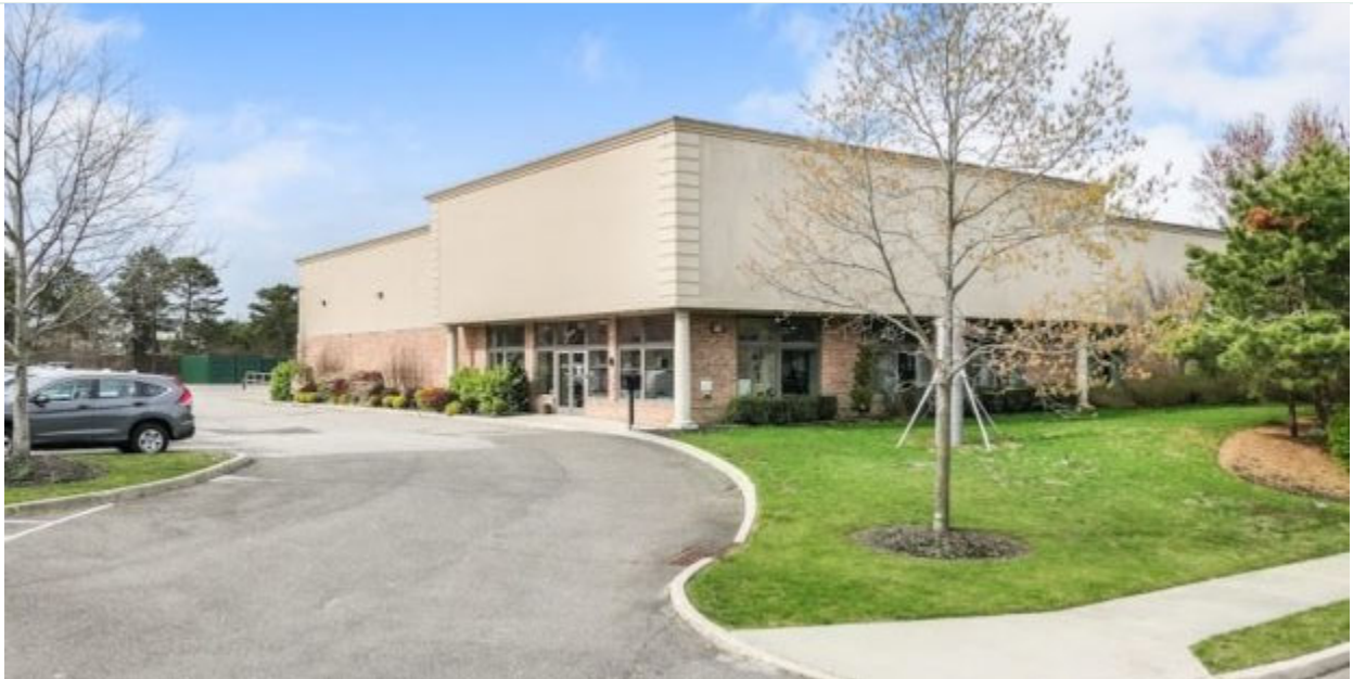
20 Pinehurst Drive Bellport / Courtesy of Douglas Elliman Commercial
